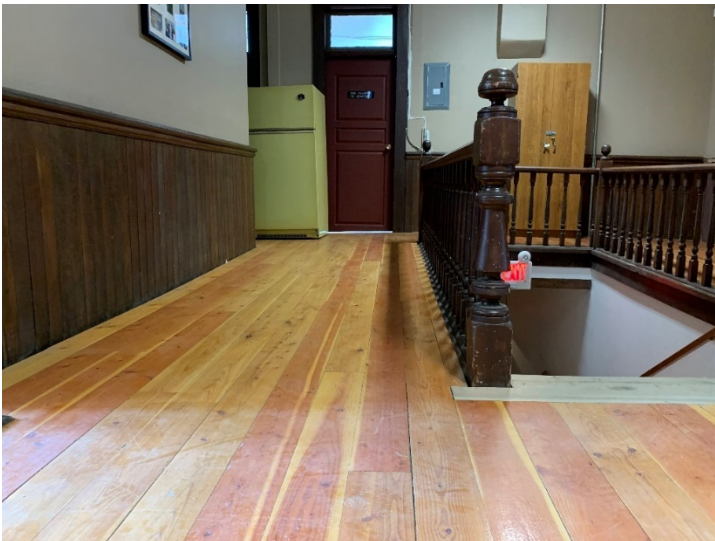
Photo 3: Stair access and flooring at second floor
