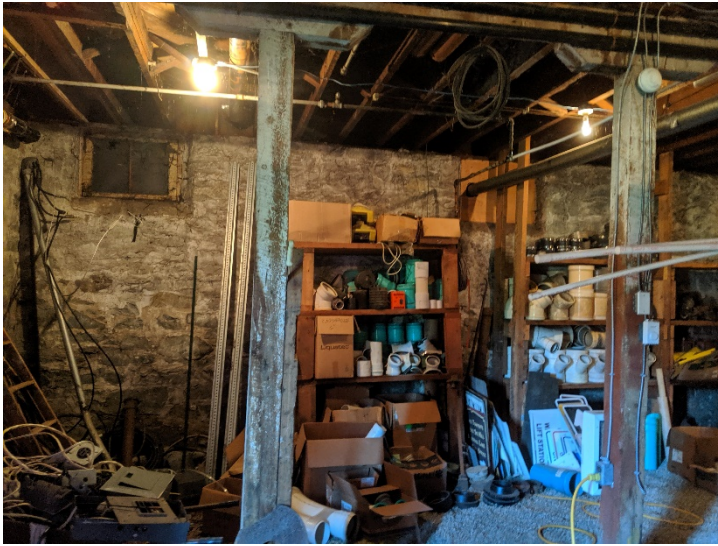
Photo 6: Basement at west side
